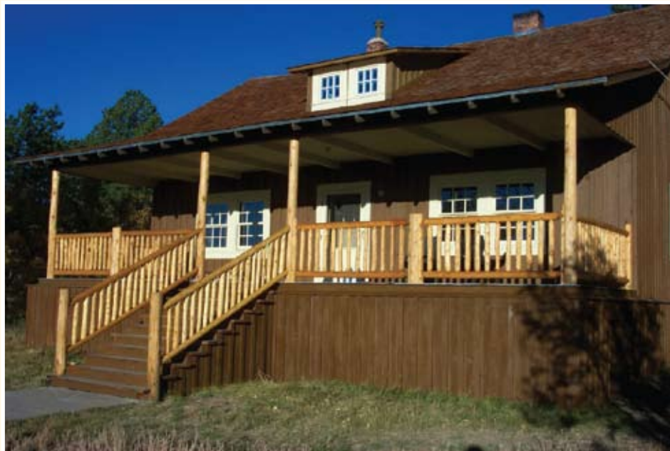
The refurbished “Mia Casita” of Aldo and Estella Bergere Leopold, 2006.
