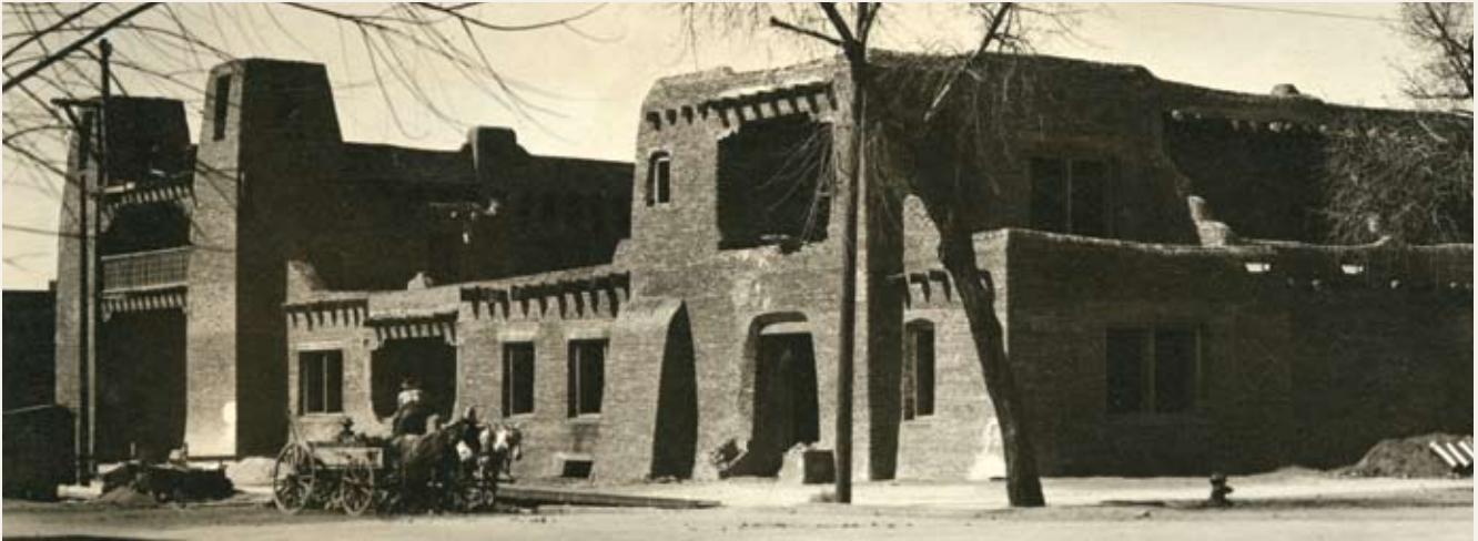
The Museum of Art under construction in 1917. Located across the street from the Palace of the Governors, the new museum would provide a much-needed venue for the rapidly expanding artist community. Courtesy of Photo Archives, Palace of the Governors (MNM/DCA), Neg. No. 012972.
